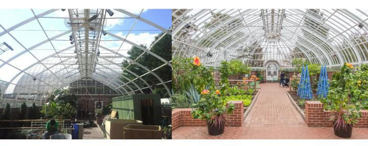
Replicated wood rafter profiles in aluminum with high performance white coating, new safety laminated glass.
