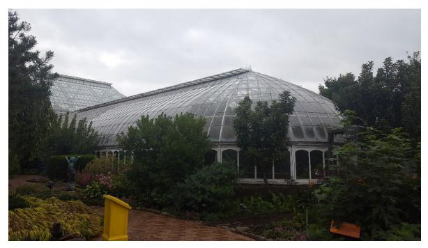
Replicated wood rafter profiles in aluminum with high performance white coating, new safety laminated glass.
