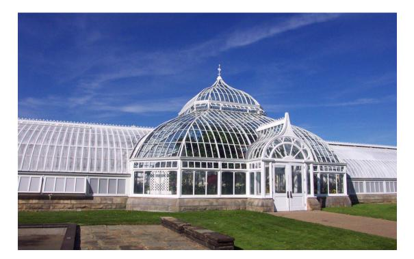
Replicated wood rafter profiles in aluminum with high performance white coating, new safety laminated glass, restored cresting and finial and automated roof vent sash.
