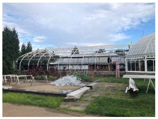
Replicated wood rafter profiles in aluminum with high performance white coating, new laminated safety glass, painting/coating of structural elements, new gutters, sills, sidewall window vents, critter screening & vent motors.
