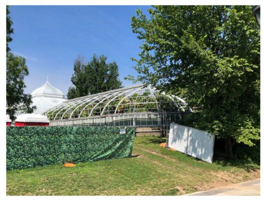
Replicated wood rafter profiles in aluminum with high performance white coating, new laminated safety glass, painting/coating of structural elements & gutters, & new insect screening & vent motors .
