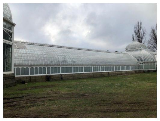
Replicated wood rafter profiles in aluminum with high performance white coating, new safety laminated glass.
