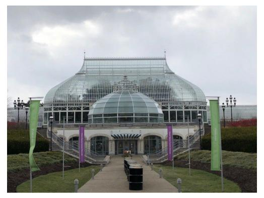
Replicated wood rafter profiles in aluminum with high performance white coating, new safety laminated glass, returned Historic Ogee Roof Structure and ornamental features.
