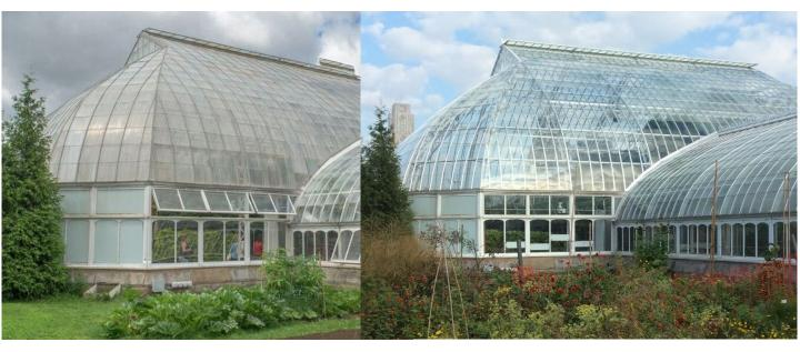
Replicated wood rafter profiles in aluminum with high performance white coating, new safety laminated glass. Return historic glass spacing, sizing and ornamental cresting ridge element.
